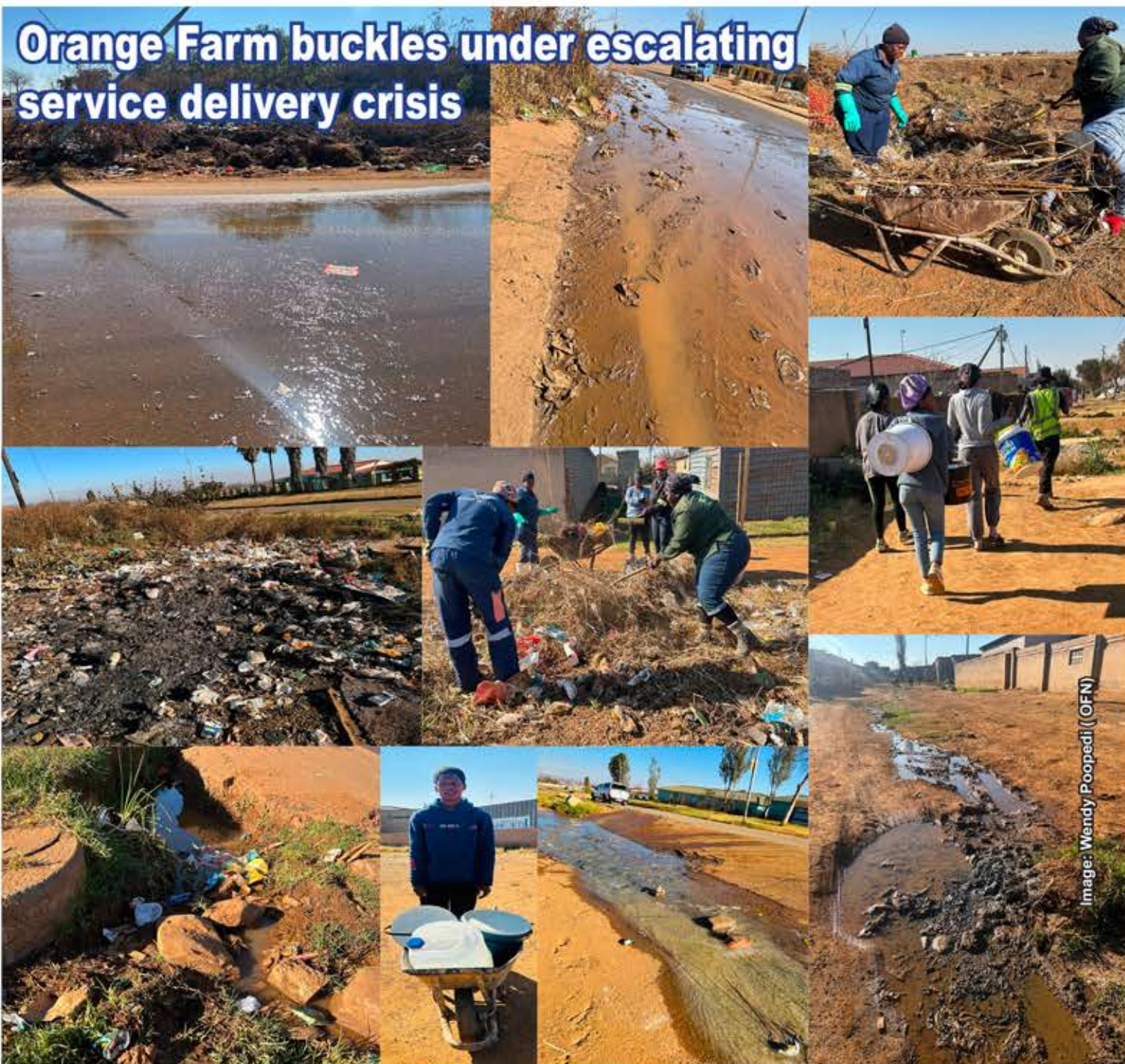
Overflowing sewerage, stagnant wastewater, illegal dumping and deteriorating roads continue to plague residents across Drieziek 1, Ext 9 Phase 1, Ext 6b, 7b, 8a and 8b. Residents say the conditions are threatening their health, safety and dignity as repeated complaints appear to have brought little lasting relief
