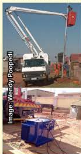
Technicians carry out transformer installation work in Ward 4 as part of ongoing electricity infrastructure
